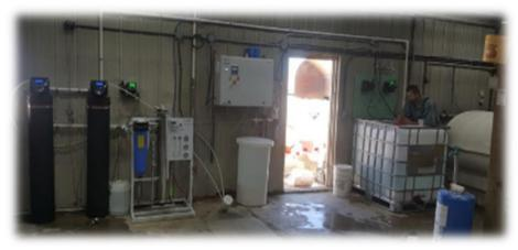
Installed an ELA-2000 Anolyte Generator to produce an Antibiotic Free Turkey operation
